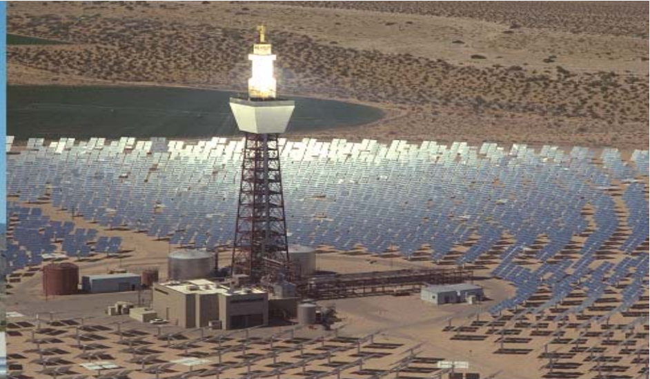
solar tower (SNL)
